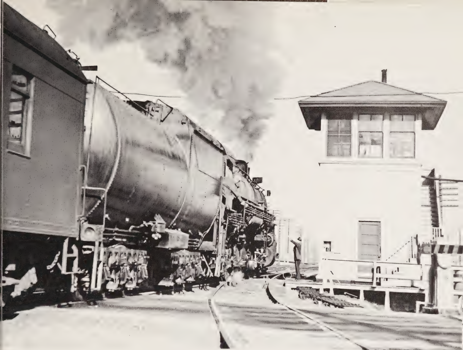
In the Grand Manner of Steam Railroading the Operator Hands the Train Order Hoop to Waiting Engineman at Burbank Junction Where the Coast Line and San Joaquin Valley Line Part Company. (LEFT) Decked in Striking Red and Orange Livery the "Coast Daylight" departs Los Angeles Union Station under a Blanket of Southern California Fog.
